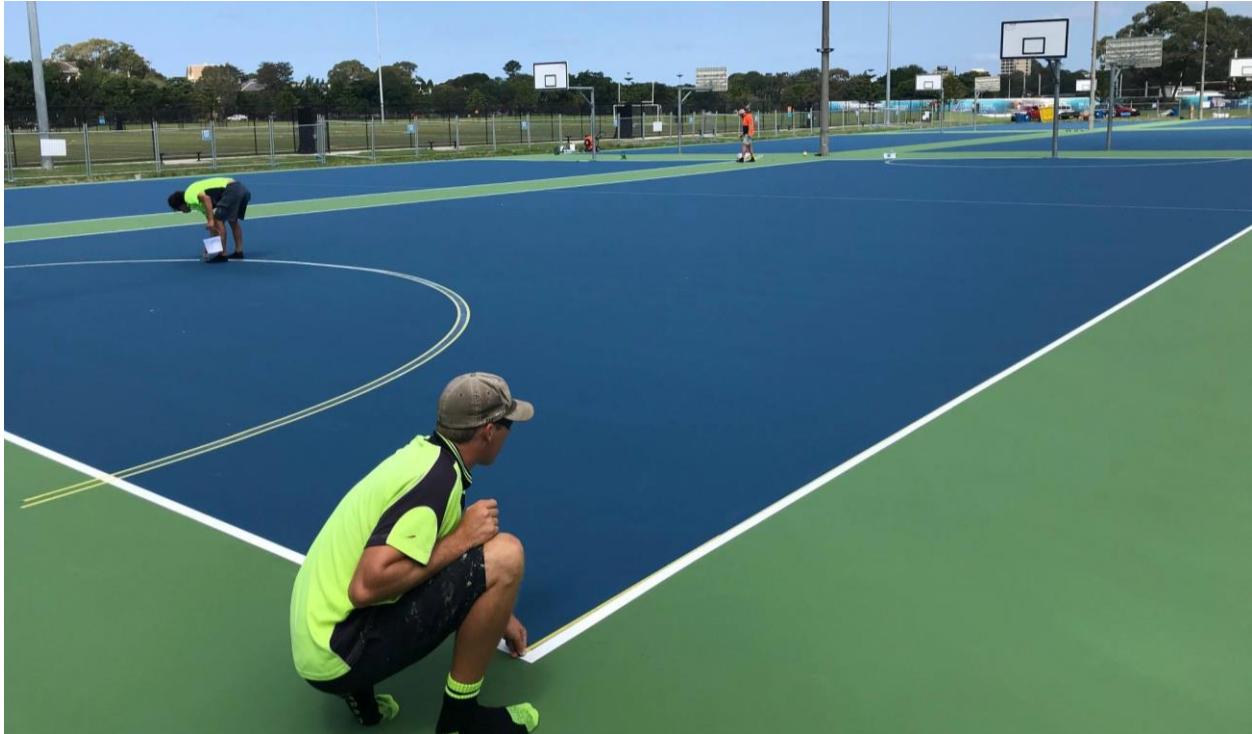
Applying line marking to basketball court
