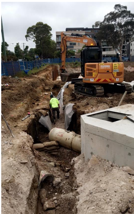
Excavation for drainage
