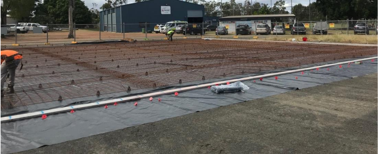
Installation of reinforcement
