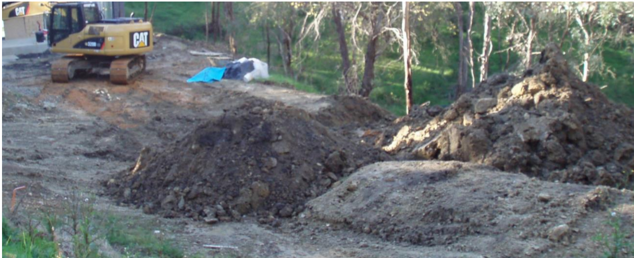
Excavating a new site
