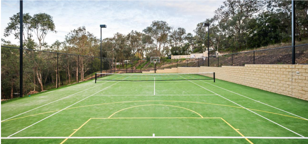
Retaining wall installed to support bank
