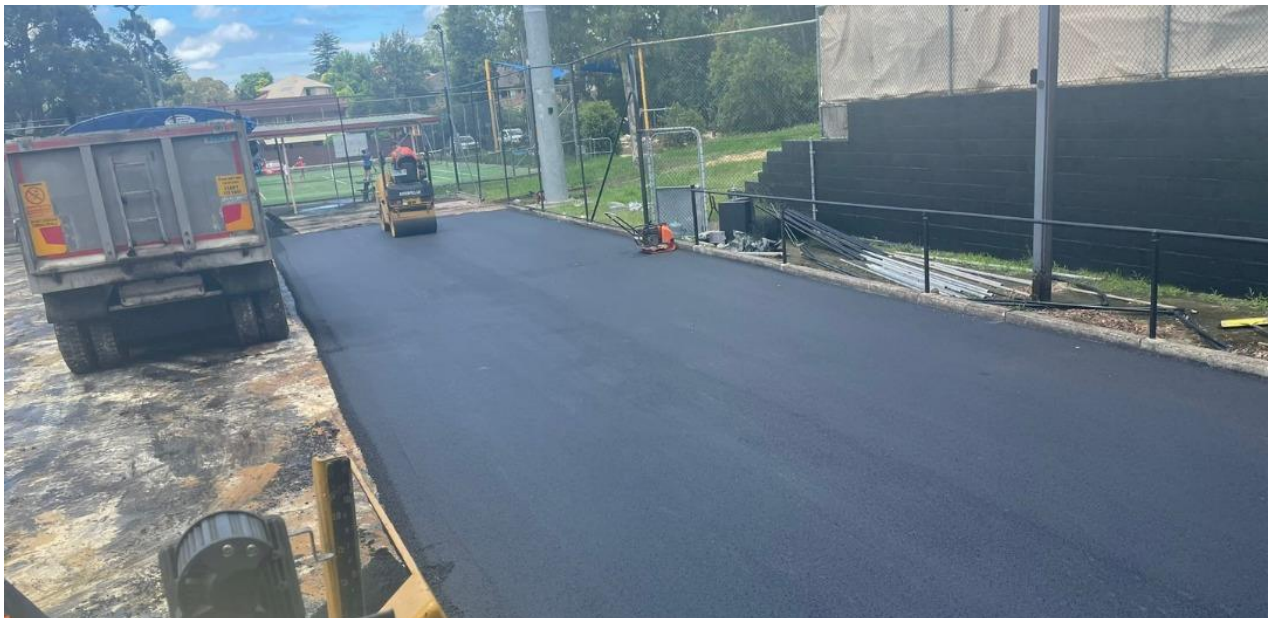
Asphalt being laid
