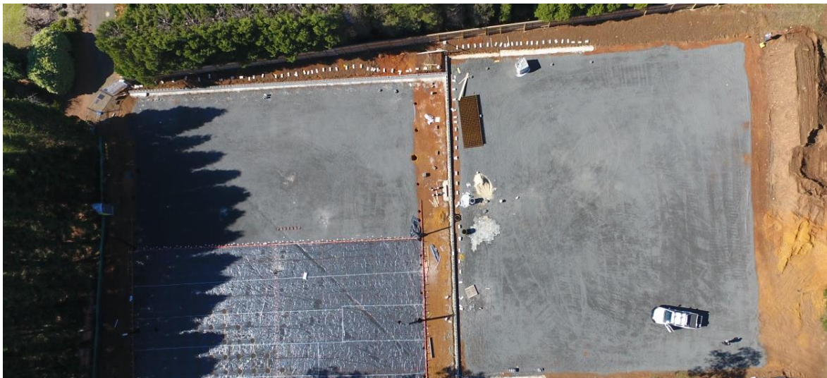
Multi-court baseworks in progress
