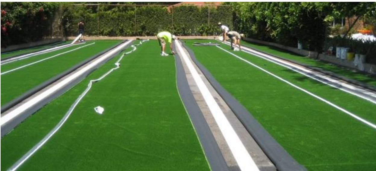
Installing a domestic synthetic grass tennis court
