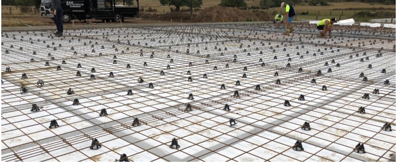
Figure 32 – Installation of alternate concrete slab design
