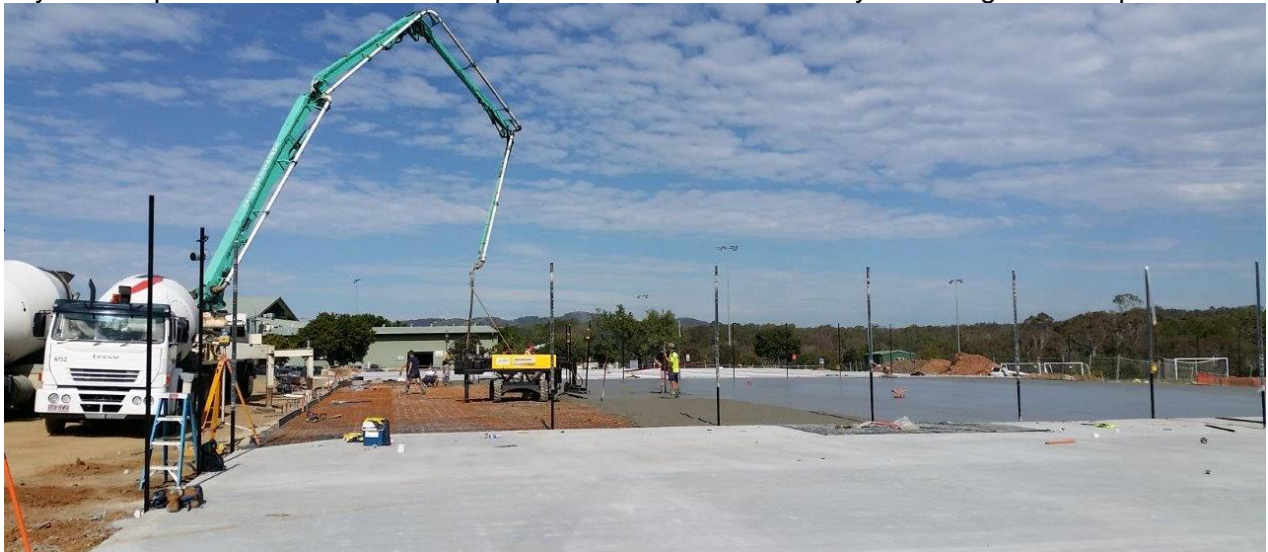
Installation of concrete
