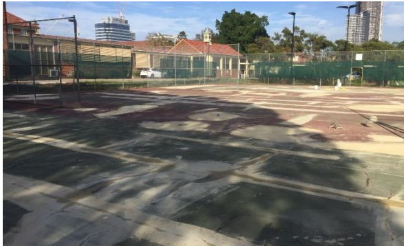
Extensive patching on old asphalt courts prior to resurfacing
