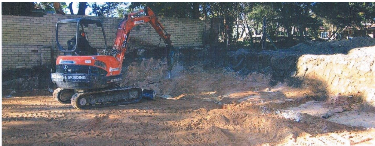
Excavation of a bank
