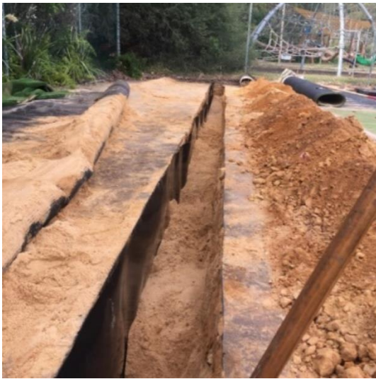
Installation of root barrier
