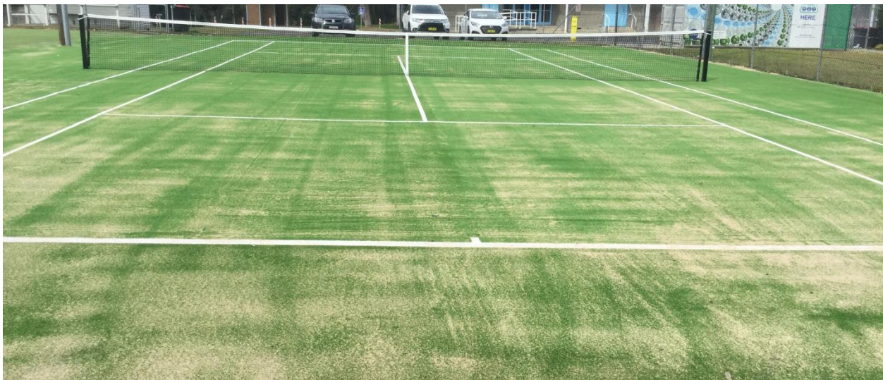
Acceptable level of sand in newly-constructed SFAG tennis court
