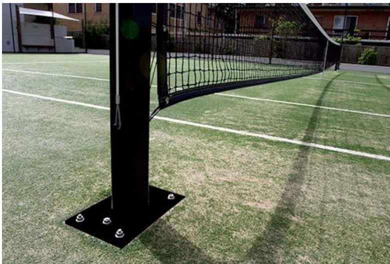
Example of common type of tennis net post baseplate mounting
