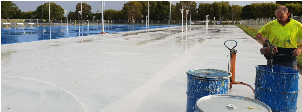
Mixing surfacing materials for netball court complex
