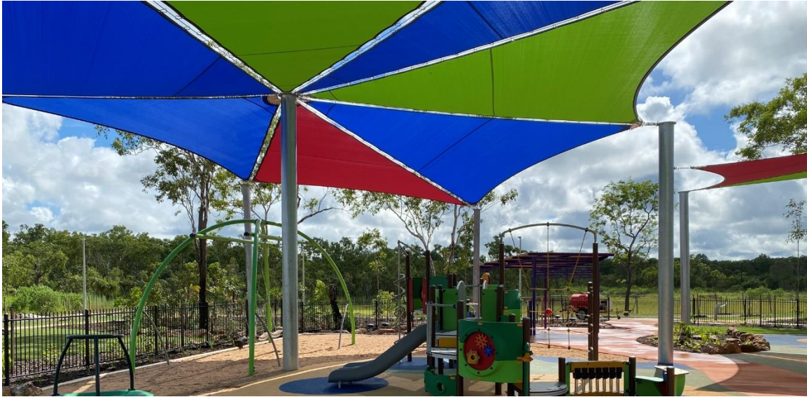
Shade structure manufactured and installed by NT Shade, Playgrounds & Rubber
