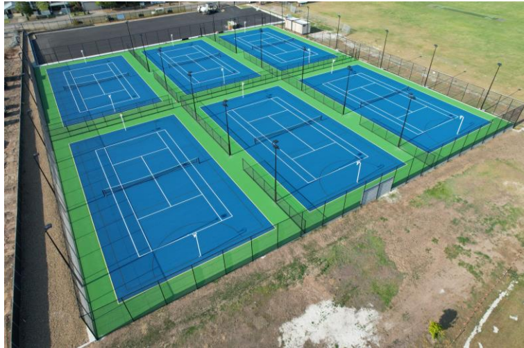
THE SPORTS COURT BUILDERS Brisbane State High School QLD
