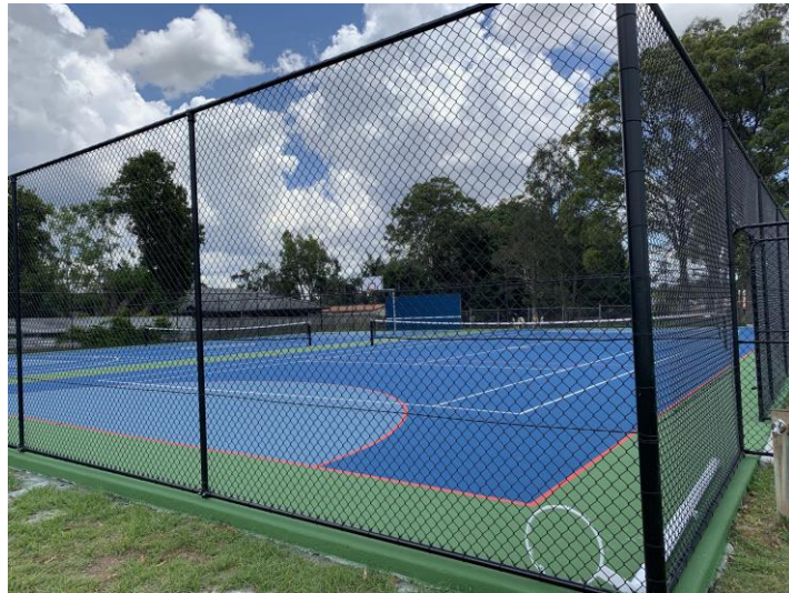
JORDIN SPORTS CONSTRUCTIONS Bray Park State School QLD
