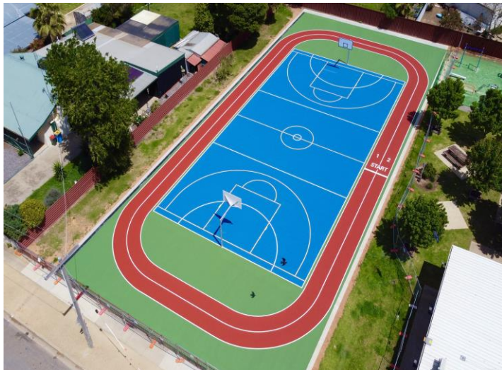
B+T POOL PAINTING + COURT SURFACING St Francis Primary School Nathalia VIC
