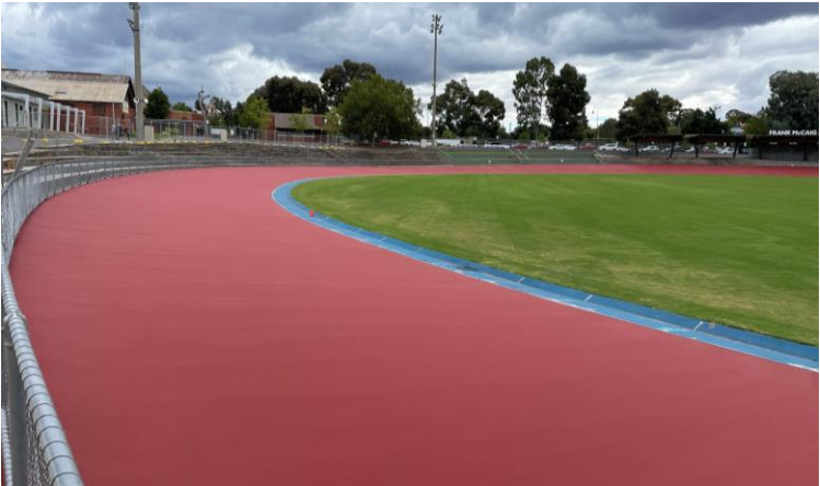
B+T POOL PAINTING + COURT SURFACING Tom Flood Sports Centre Velodrome VIC
