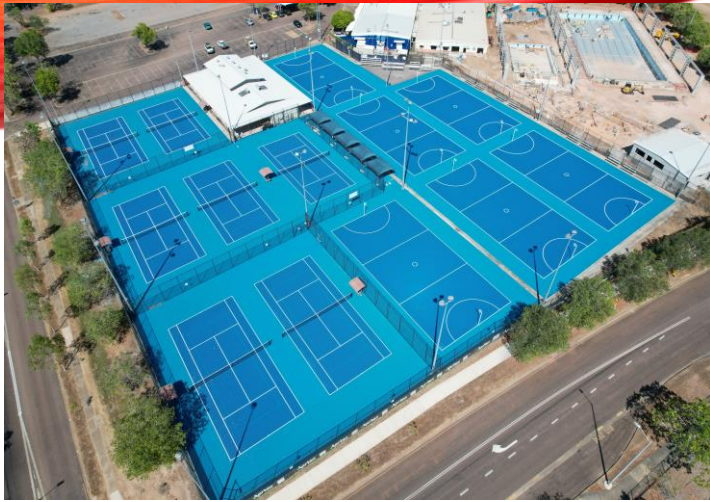
THE SPORTS COURT BUILDERS Palmerston Tennis/Netball Darwin NT
